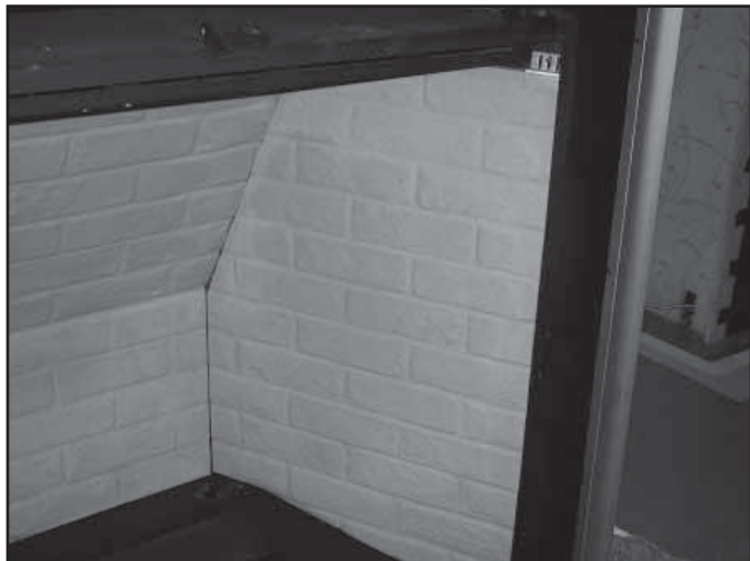
Figure 15.4 Install Right Side Refractory
